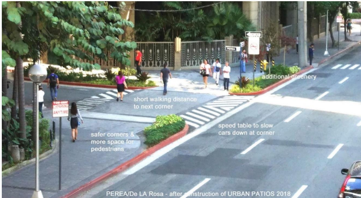
Figure 34. Example of a well-designed junction which reduces the potential for poor driving behaviour.
