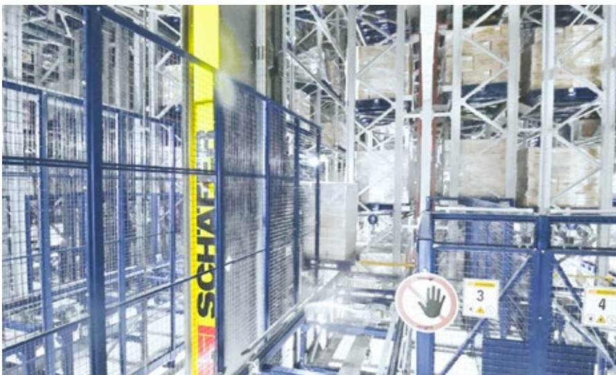
Operating in a seismic zone, the ORCA 45-meter-high facility was built with a rack-clad designed structure.
