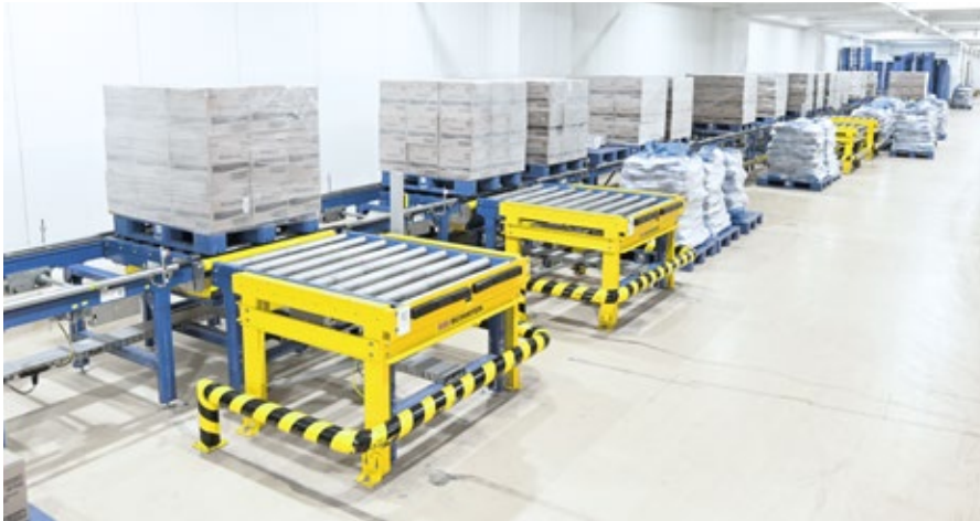
The 282-meter long conveying system connecting to key individual areas of the warehouse.
