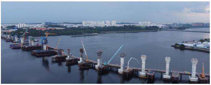
A railway viaduct is taking shape across the Strait of Johor. A trestle bridge has also been erected.
